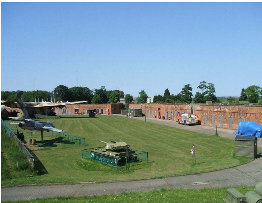
Paul Point after restoration
